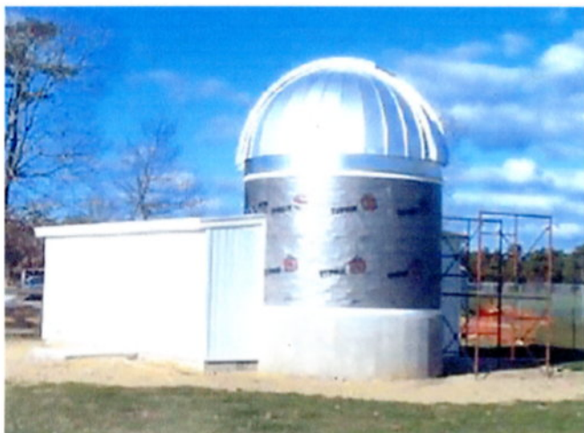
The Schmidt nearing completion
